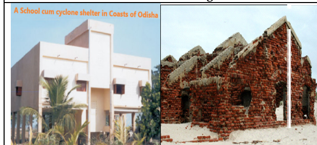
Fig 3: (A) Recently constructed cyclone shelter (B) Eroded post SuCS 1999 in JSPurOdisha, without care Source: https://www.thestatesman.com/cities/coastal-villages-jagatsinghpur
