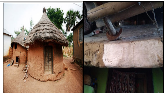
Fig 2 : (A) Attu portion visible (b) Traditional informal storm resilient houses in tribal villages of Odisha
