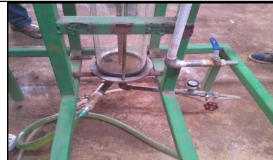
Fig. 8 Bottom section of the scrubber
