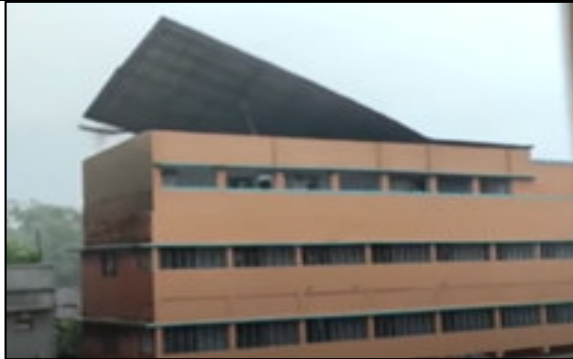
Fig 5 :The roofblown away during ESCS Amphan in Kolkata 21 st May 2020
